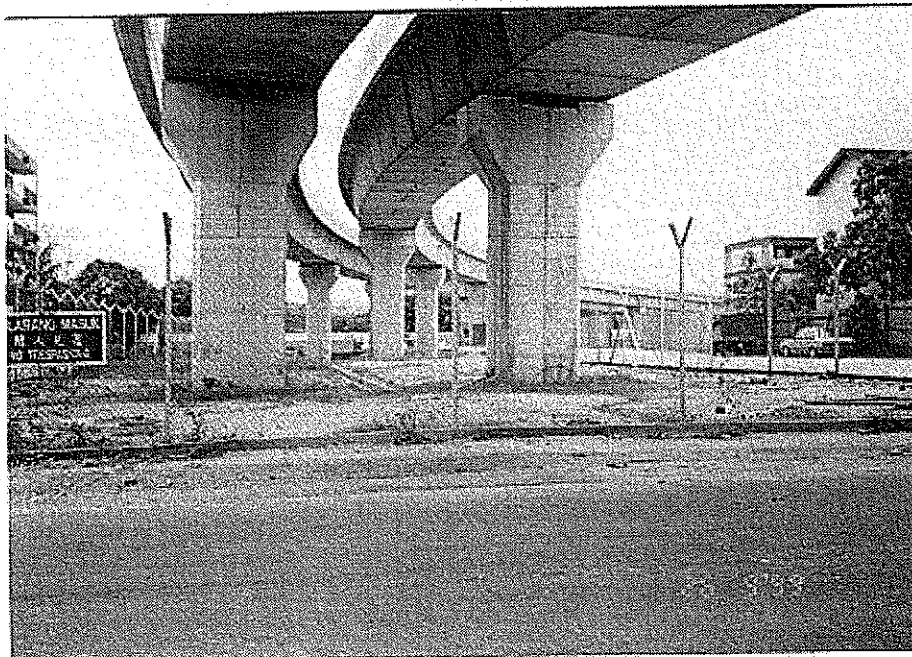
HO HUP CONSTRUCTION CO. - LRT 2 For Kuala Lumpur Section 2B/2C Damai Portal To Gombak Terminal Pilecaps & Piers Construction
