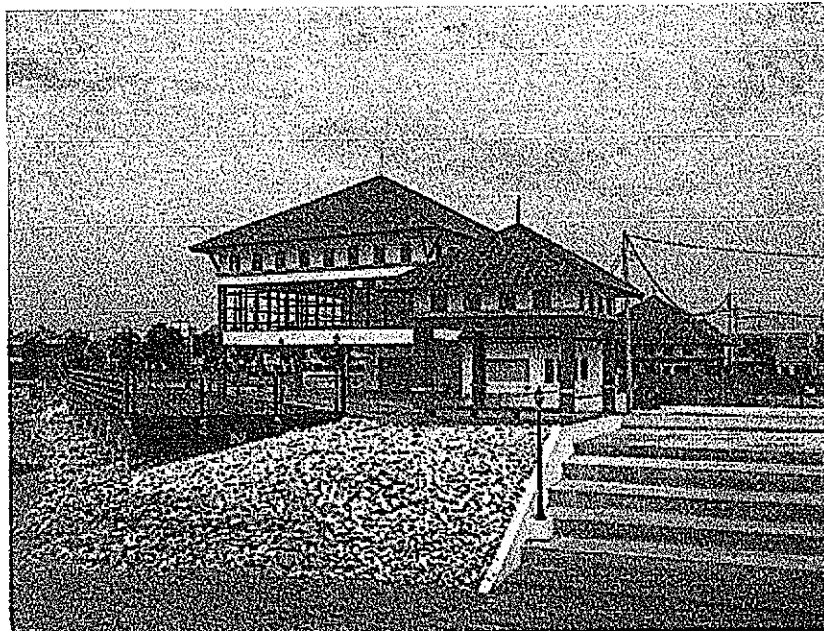
Cadanagan Pembina Jeti Secara Build, Operate and Transfer (B.T.O) Di Seksyen 10, Pulau Indah (KS7) Klang Diraja, West Port
